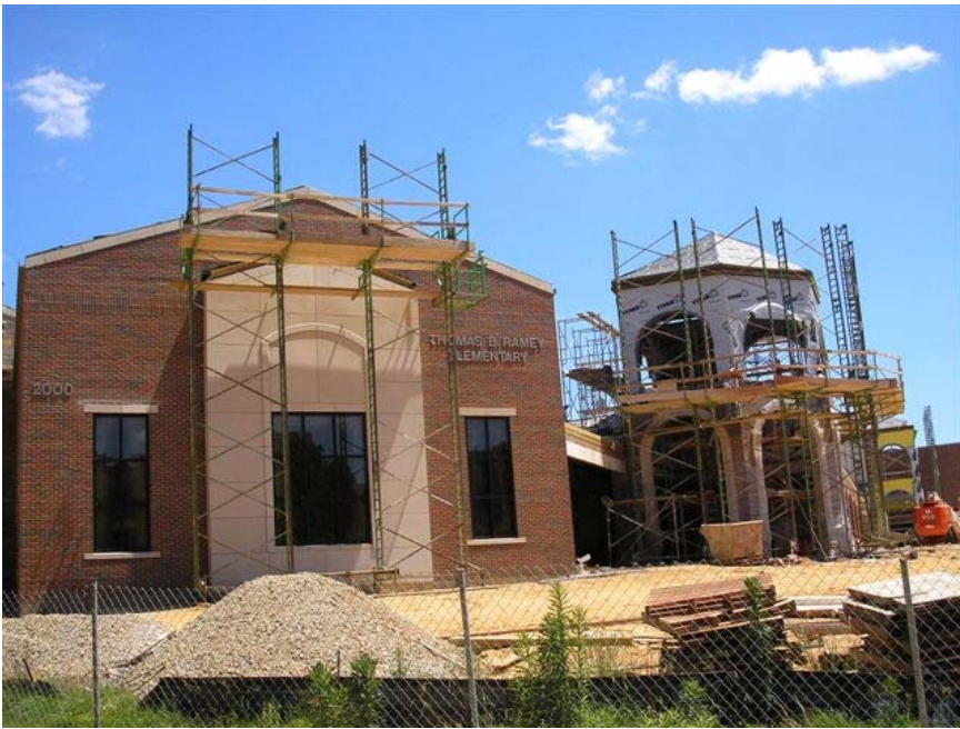
Bell Elementary Construction Photos - May 2006
