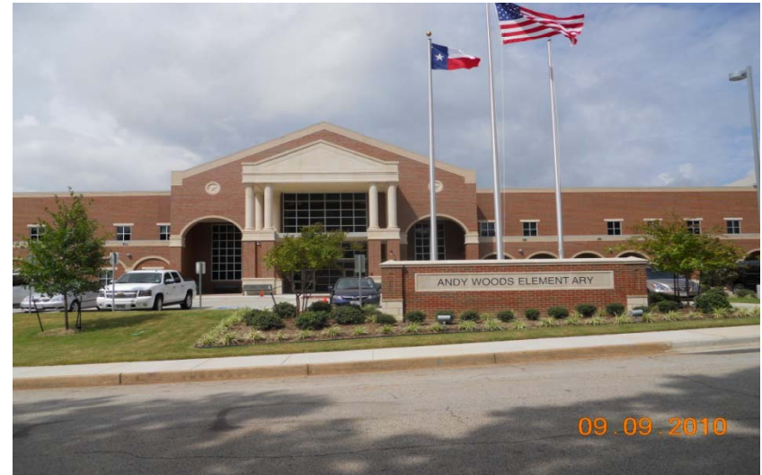
Photo #4 Andy Woods Elementary 9-09-10 East (Front ) Elevation
