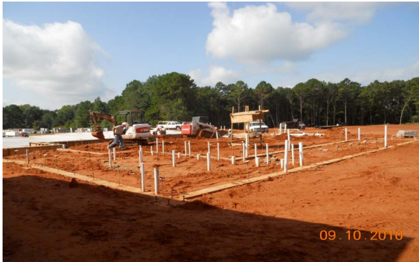
Photo #3 Prep for Gym Slab
