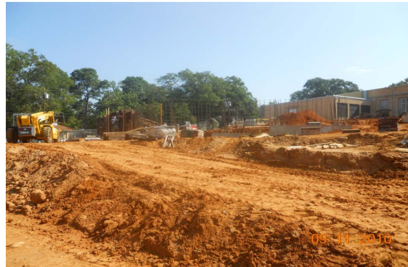
Photo #6 Birdwell Elementary 9-11-10 New Gym/Cafeteria Area
