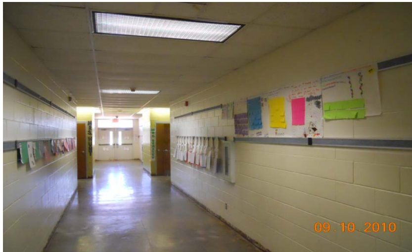
Photo #7 Owens Elementary 9-10-10 Existing Corridor
