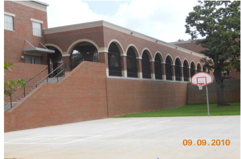
Photo #2 Andy Woods Elementary 9-09-10 Stairway From Walkway to Play Court
