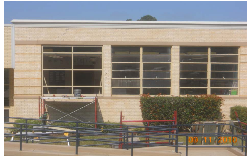
Photo #8 Birdwell Elementary 8-13-10 New Window on Left Old on Right
