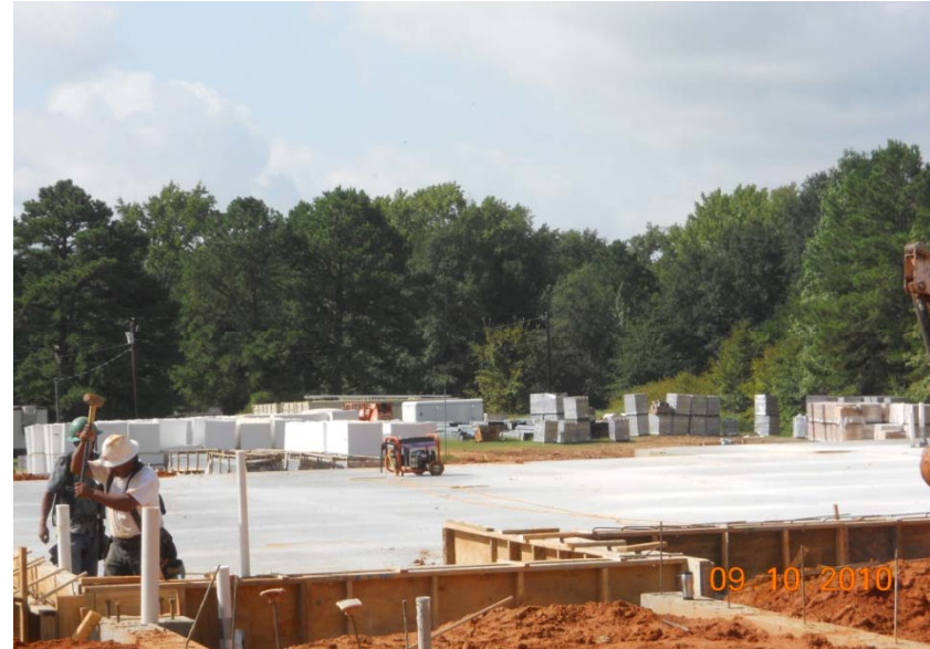
Photo #2 Cafeteria Slab
