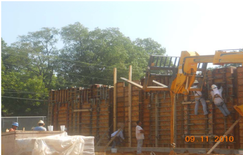
Photo #7 Birdwell Elementary 9-11-10 Foundation Walls at Gym
