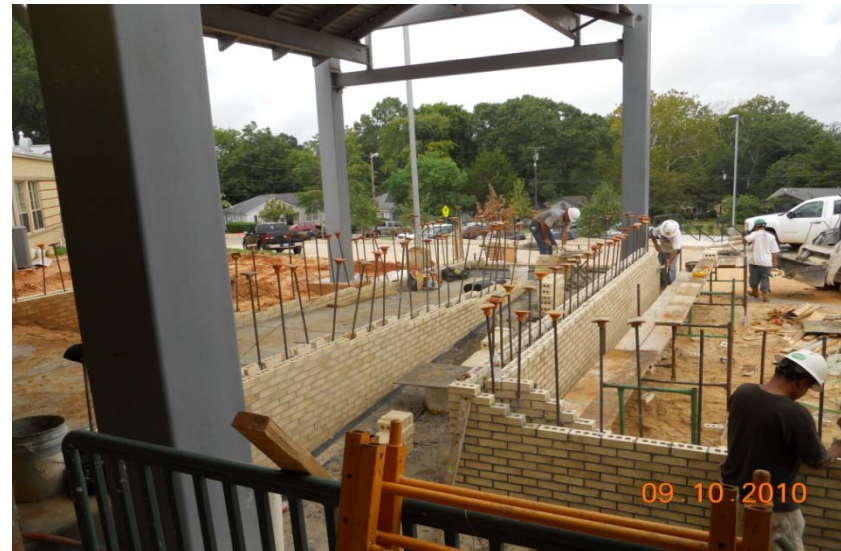
Photo #2 Handicap Ramp At New Entry
