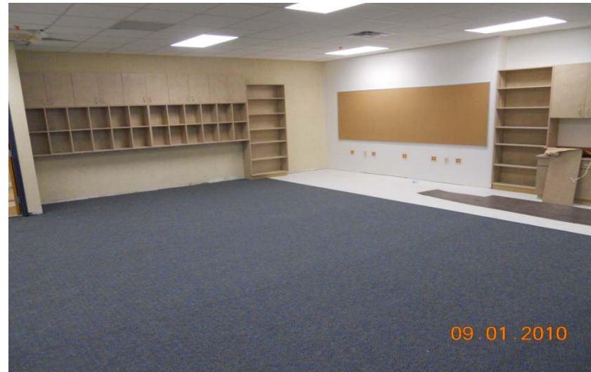
Photo #4 Completed Classroom
