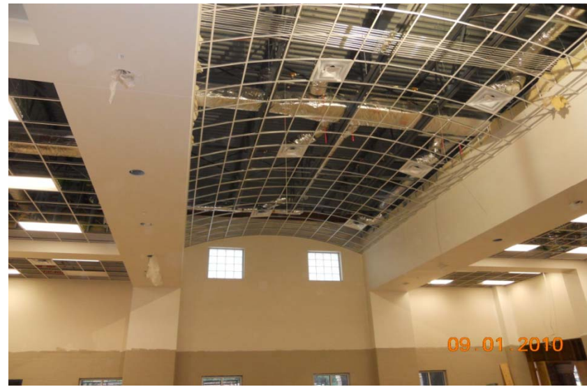
Photo #2 Cafeteria Ceiling
