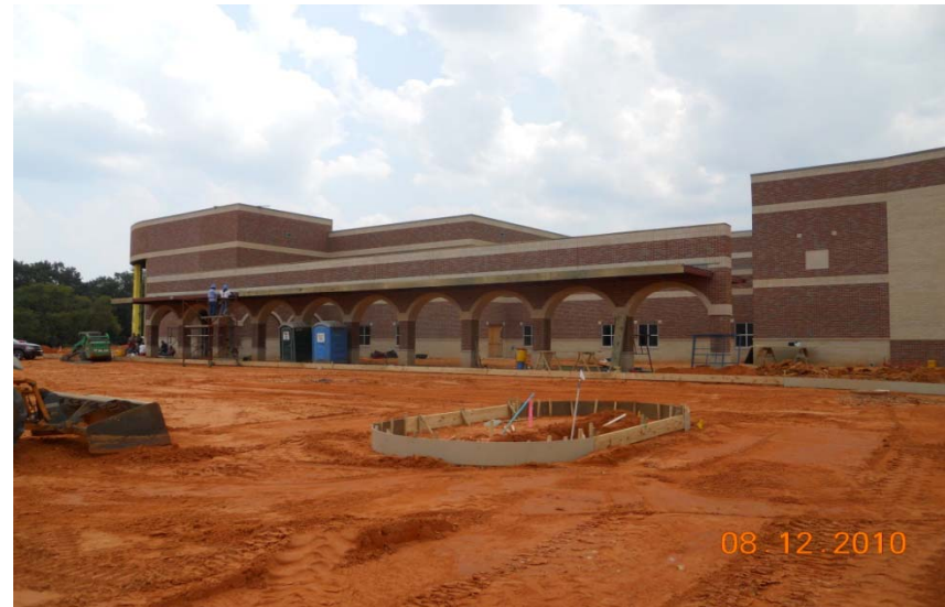
Photo #2 West Elevation
