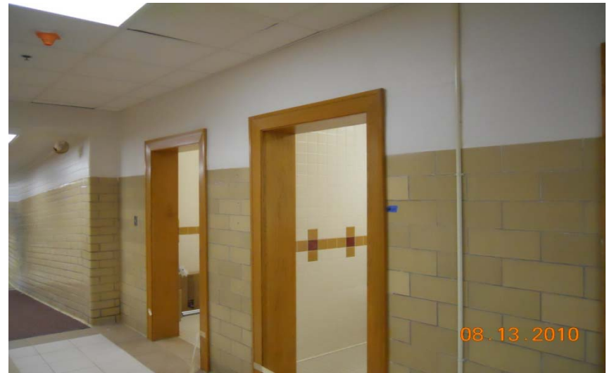
Photo #4 Birdwell Elementary 8-13-10 Classroom Corridor
