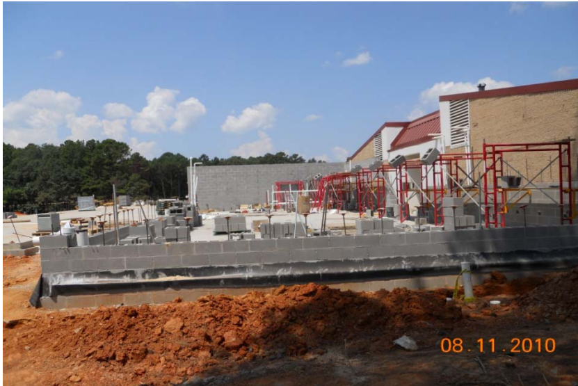
Photo #1 Owens Elementary 8-11-10 New Classroom Addition
