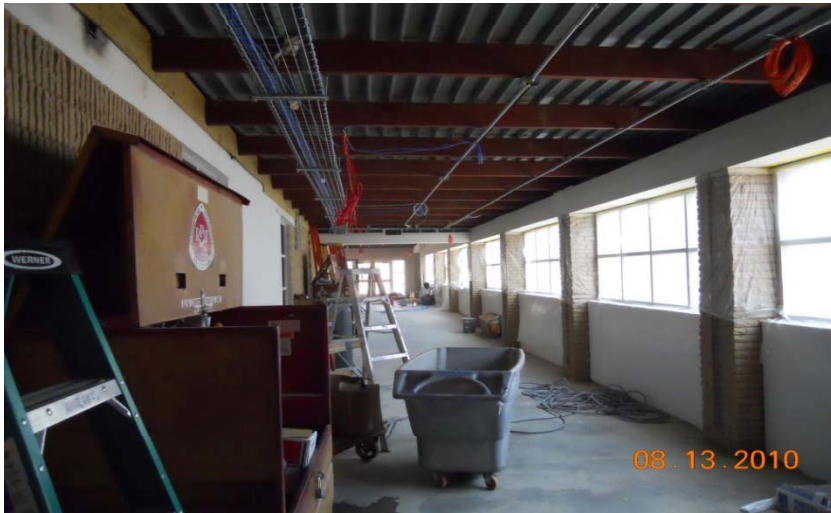
Photo #3 Owens Elementary 8-13-10 New Connecting Corridor
