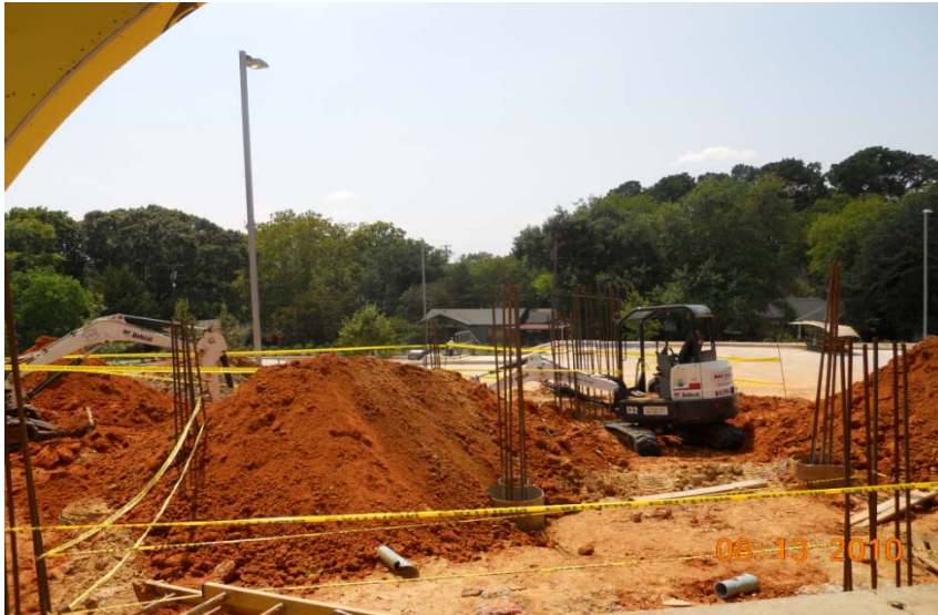
Photo #1 Birdwell Elementary 8-13-10 Foundation at New Gym
