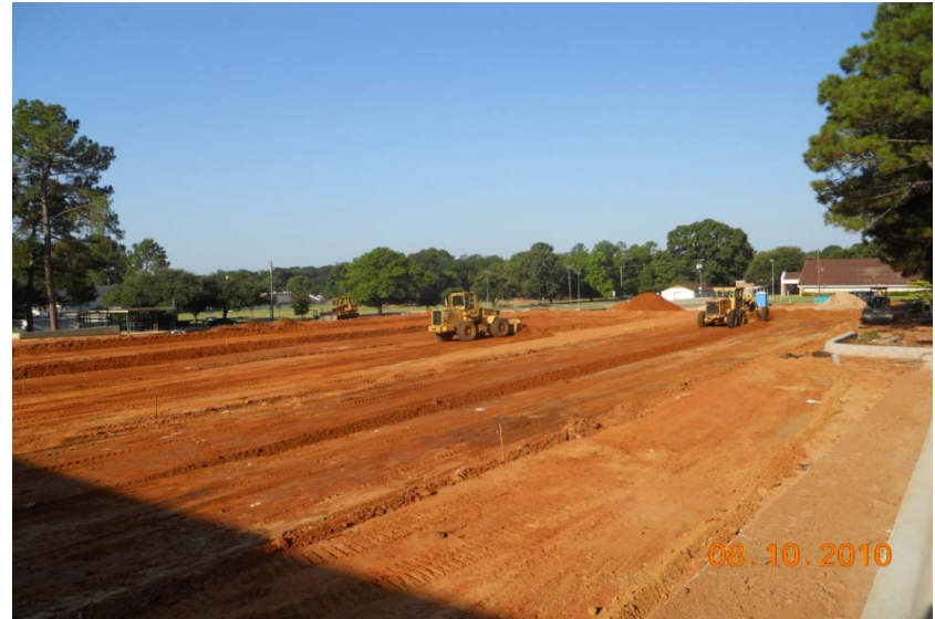
Photo #2 Grading at New Play Area
